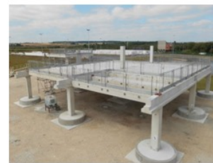
Photo 2: M-Frame delivered at Explore Manufacturing P88 Demonstrator
